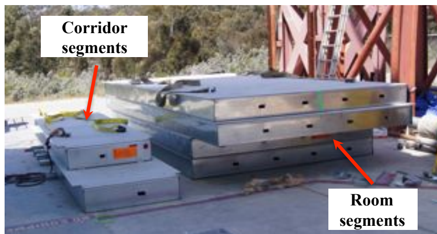
Figure 2.10. Diaphragm panel pattern (top) and photographs of the prefabricated diaphragm segments prior to installation (bottom) (room segments #1 – #4 and corridor segments #5 and #6).
