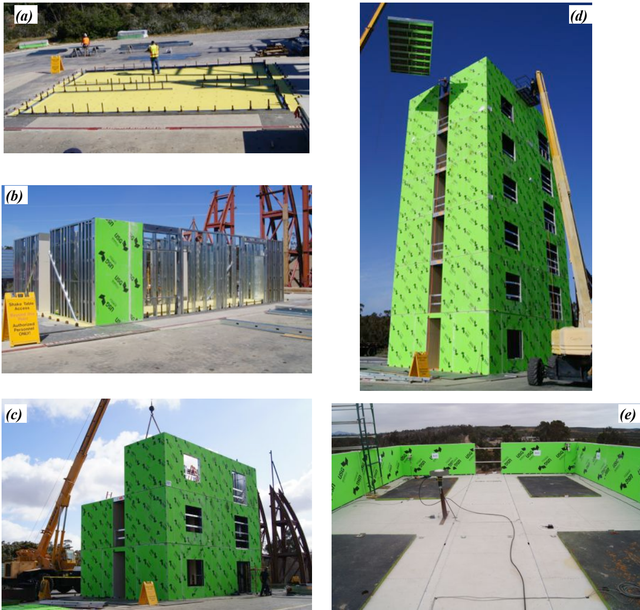
Figure 2.12. Construction of the test building: (a) building tie-down system (photo taken on April 16, 2016), (b) in-situ installation of first-story wall system (photo taken on April 19, 2016), (c) installation of a prefabricated wall panel at the third story (photo taken on April 23, 2016), (d) completion of building skeleton erection (hoisting the last piece of roof panel) (photo taken on April 27, 2016), and (e) roof mass plate layout prior to the earthquake tests (photo taken on June 10, 2016).
