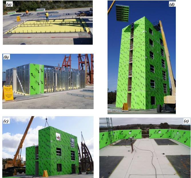
Figure 4. Construction of the test building: (a) building tie-down system (April 16, 2016), (b) in-situ installation of first-story wall system (April 19, 2016), (c) installation of a prefabricated wall panel at the third story (April 23, 2016), (d) completion of building skeleton erection (hoisting the final piece of roof panel) (April 27, 2016), and (e) roof mass plate layout prior to the earthquake tests (June 10, 2016).
