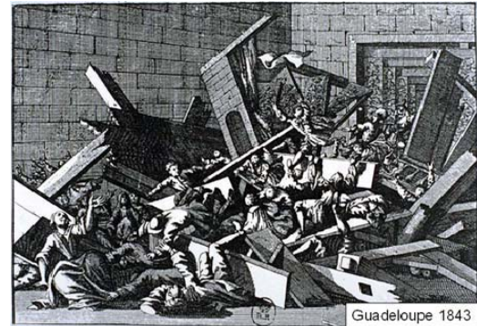
Fig. 2 Cartoon depicting observed building interior damage from the 1843 Guadeloupe earthquake. (Source: NISEE, 2009)
