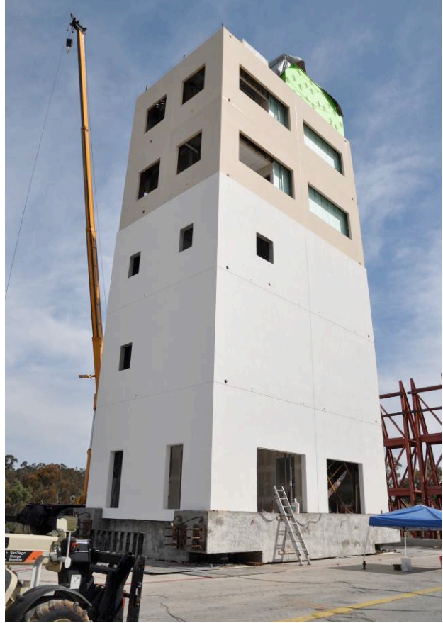
Photographs of (left) structural skeleton during façade installation (North & West elevation) and (right) completed building façade (West and South elevation) at the NEES@UCSD shake table.
