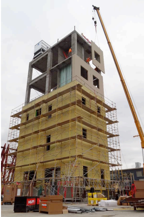
Photographs of (left) structural skeleton during façade installation (North & West elevation) and (right) completed building façade (West and South elevation) at the NEES@UCSD shake table.
